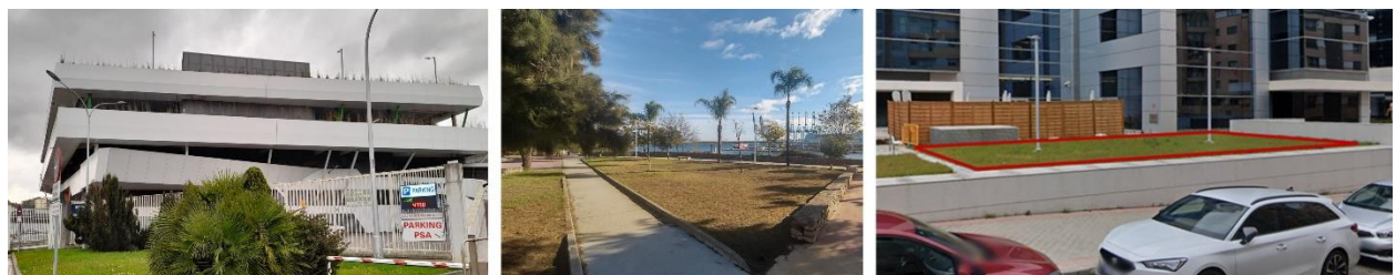
Locations of the parking lot building at Vigo (left), Plot in boardwalk in Algeciras (centre), and plot at the street level in the Aqualia Corporate Offices in Madrid (right)
