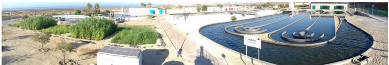
Figure 1. Panoramic view of the demonstration plant at El Toyo WWTP (Almería).
